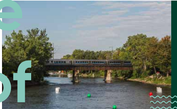
Railway bridge in Laval
