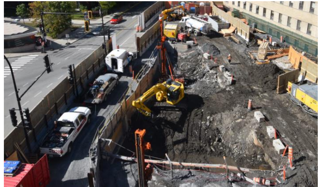
September: Drilling begins to prepare for controlled blasting
