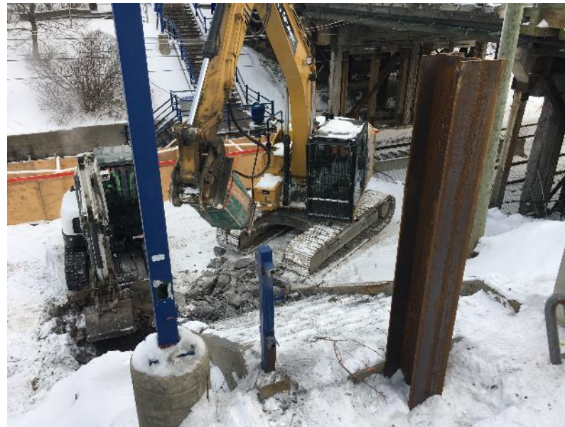
Platform and stairwell demolition at Mont-Royal
