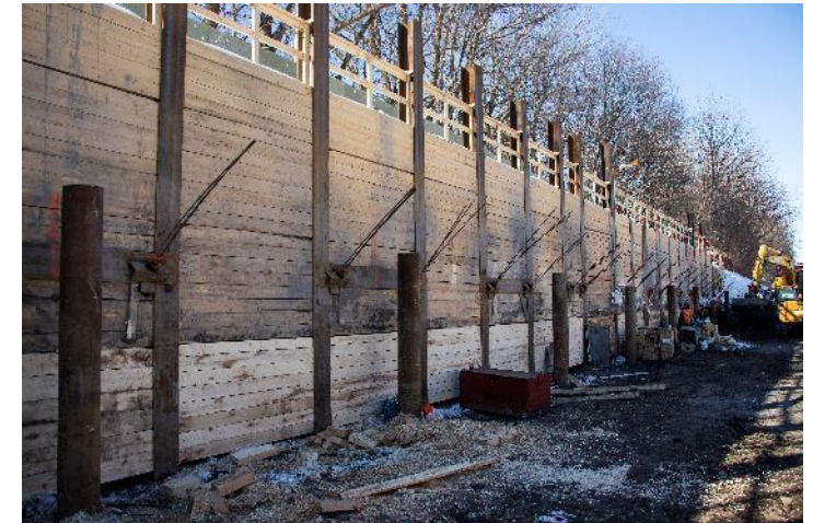
Anchoring of the retaining wall
