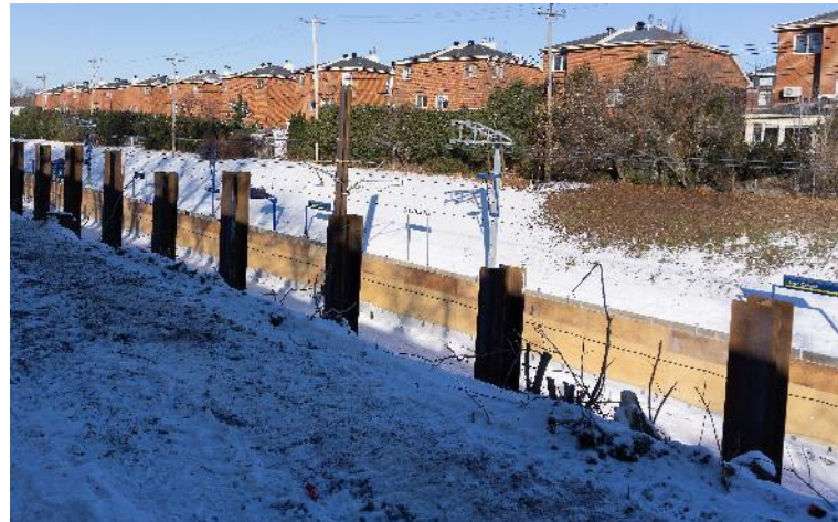
Vibratory driving and traditional driving of piles for the retaining walls
