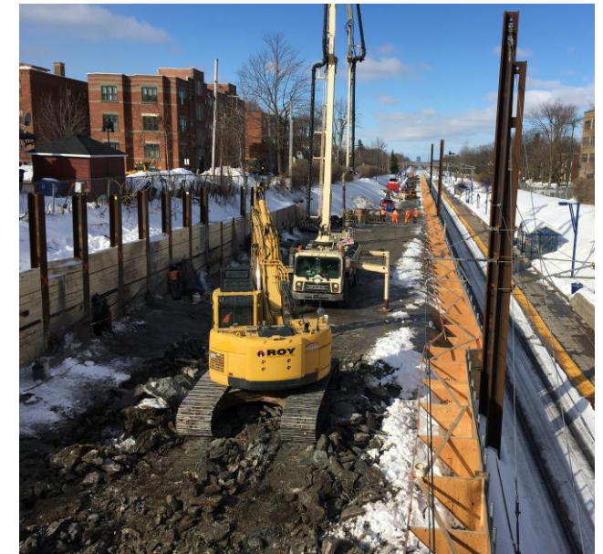
Excavation and construction of retaining walls
