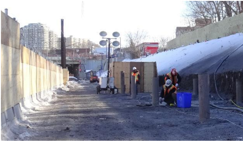
Station pile driving
