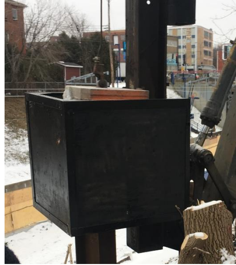
Acoustic box around hammer du virbo-sinking of piles
