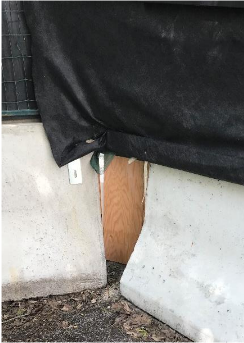
Sealed joints between jerseys
