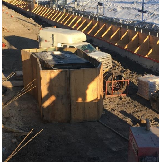
Acoustic box installed around a compressor
