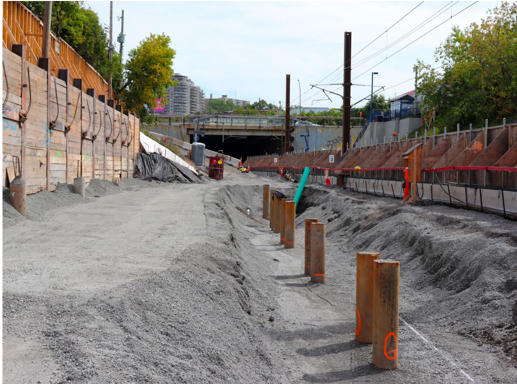
Drilling of foundation piles Canora east
