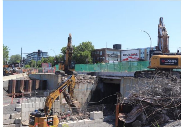
July 2020 – Demolition of the deck on the north side of the Jean-Talon Bridge
