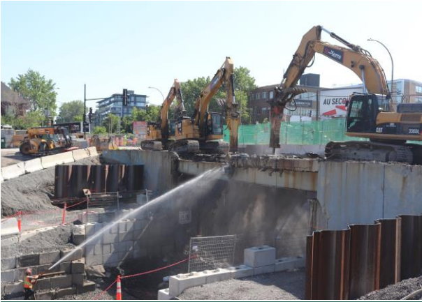
July 2020 – Demolition of the deck on the north side of the Jean-Talon Bridge
