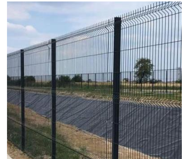
New intrusion-control fence
