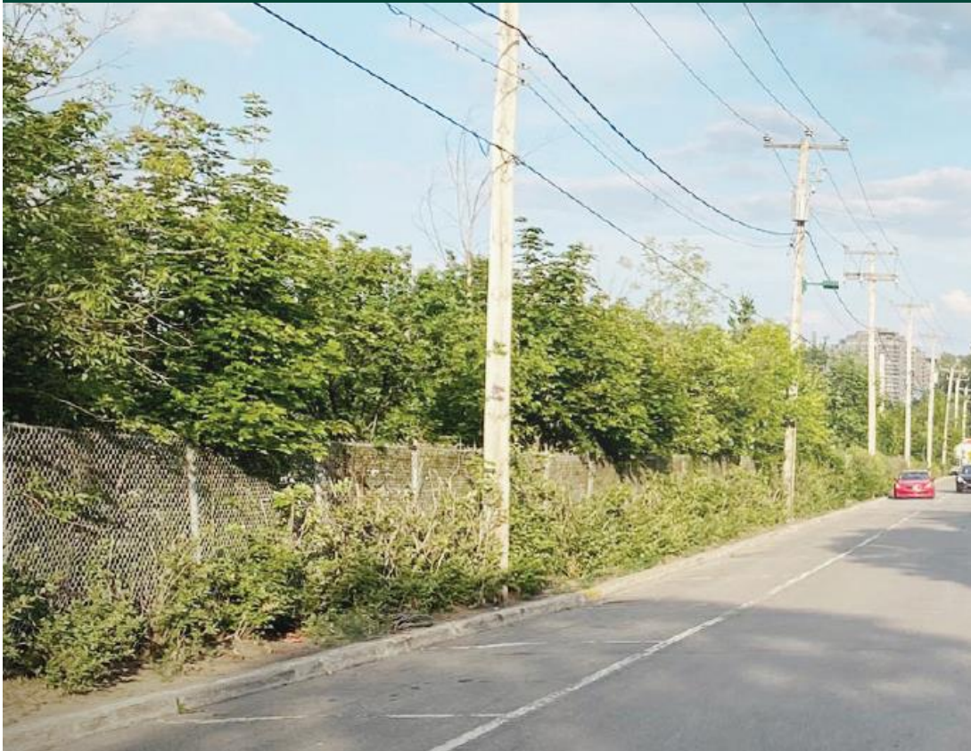
Initial status before cutting
