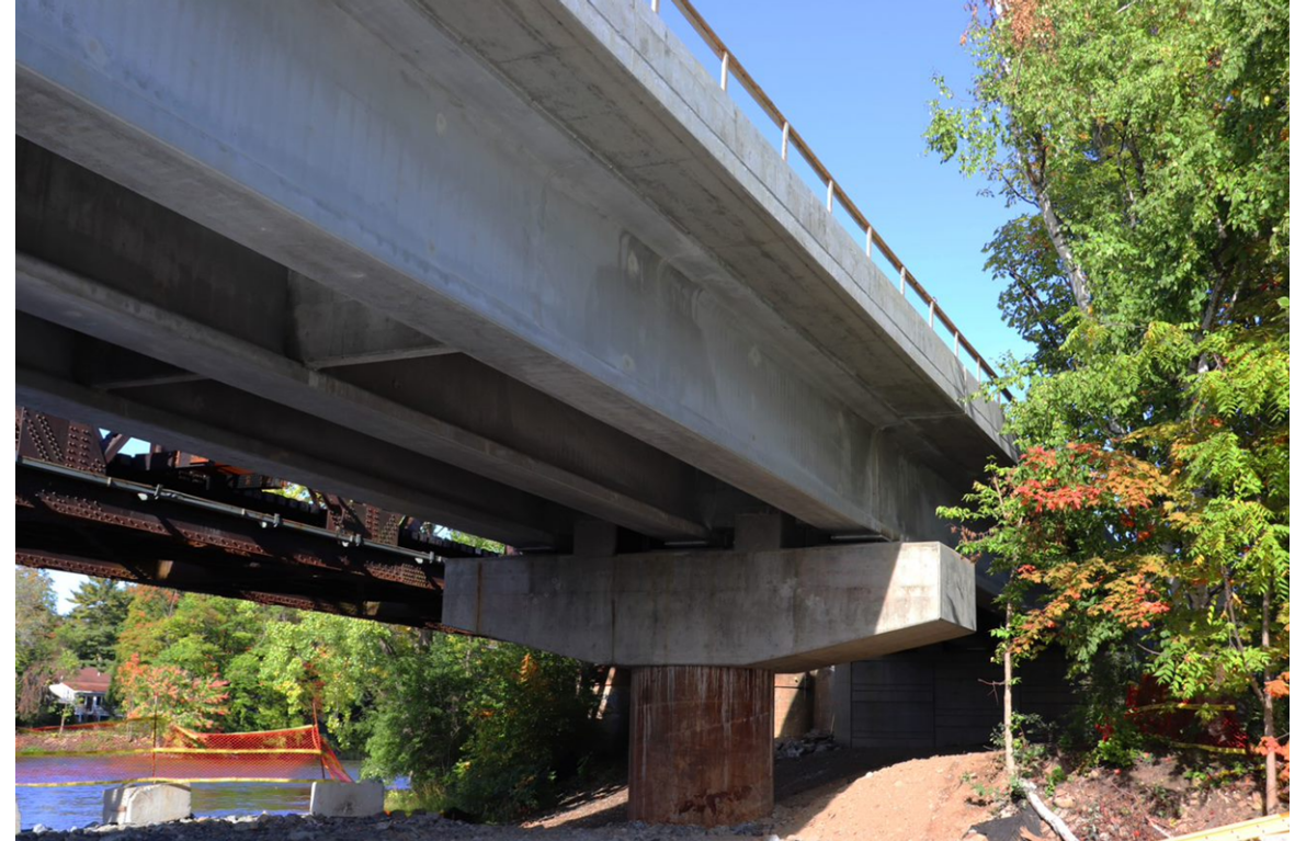
View “under” RDP1
