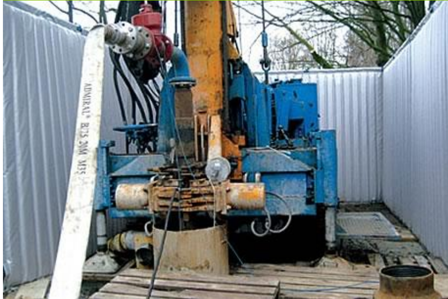
Acoustic screen for bored piles
