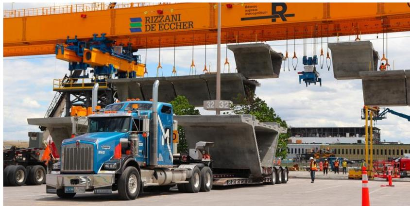
3. Concrete segments are re-assembled on the launching beam to build the spans
