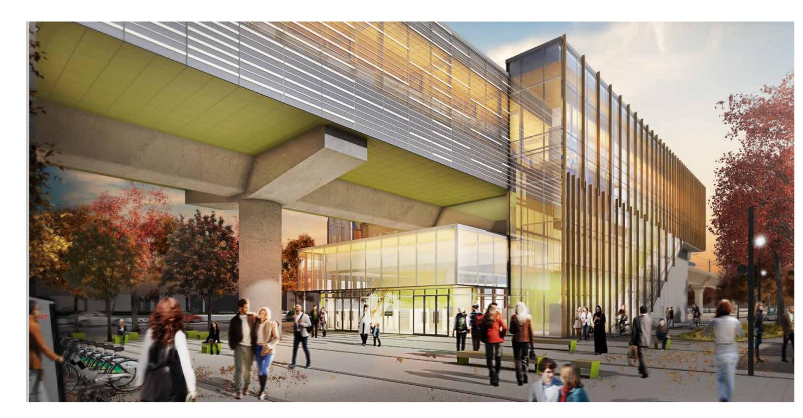
In order to let in as much natural light as possible and for increased safety, the stations are transparent (the concept of seeing and being seen). Fritted glass is used to filter the light.
